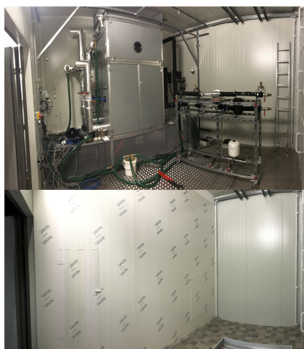
Fig. 2. Indoor space before and after installation of separation wall.
